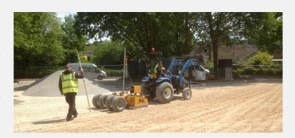
The X-Grid was laid on top of a well screeded sand blinding layer and filled with a robust decorative gravel.
